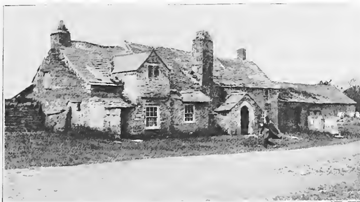
Houses Roofed with Stone
